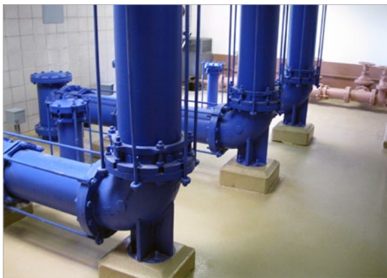
CSI Division 9: Flooring - Fluid Applied
